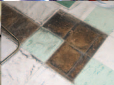
Laying new and safer flooring
